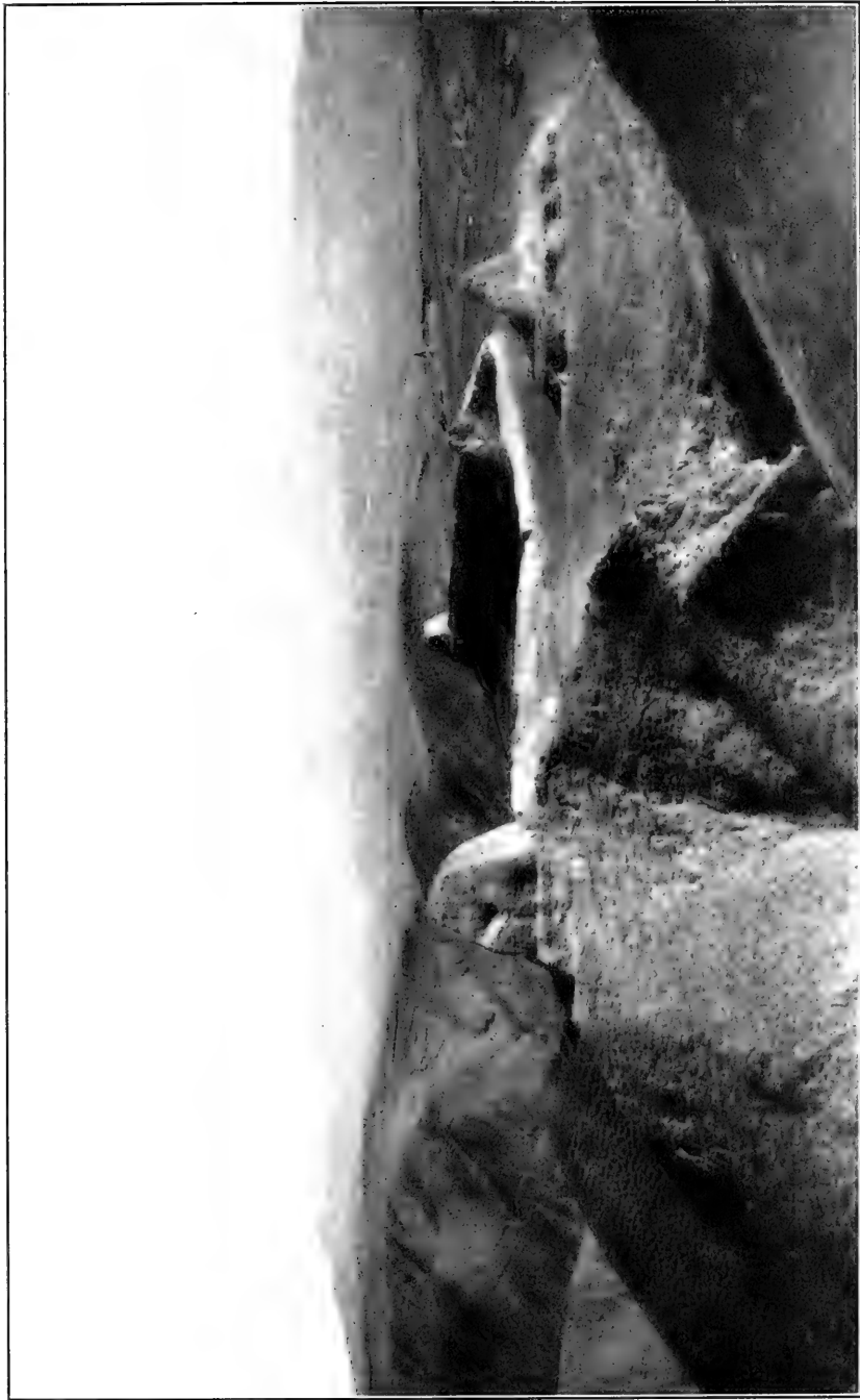
PORTION OF GREAT WALL OF CHINA, NORTHWEST OF PEKING, BUILT OF EARTH WITH EARTHEN TOWERS.
